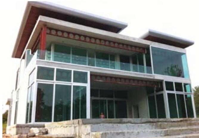
Phoenix Villa: First villa built in Thailand with long-span cellular structure.
