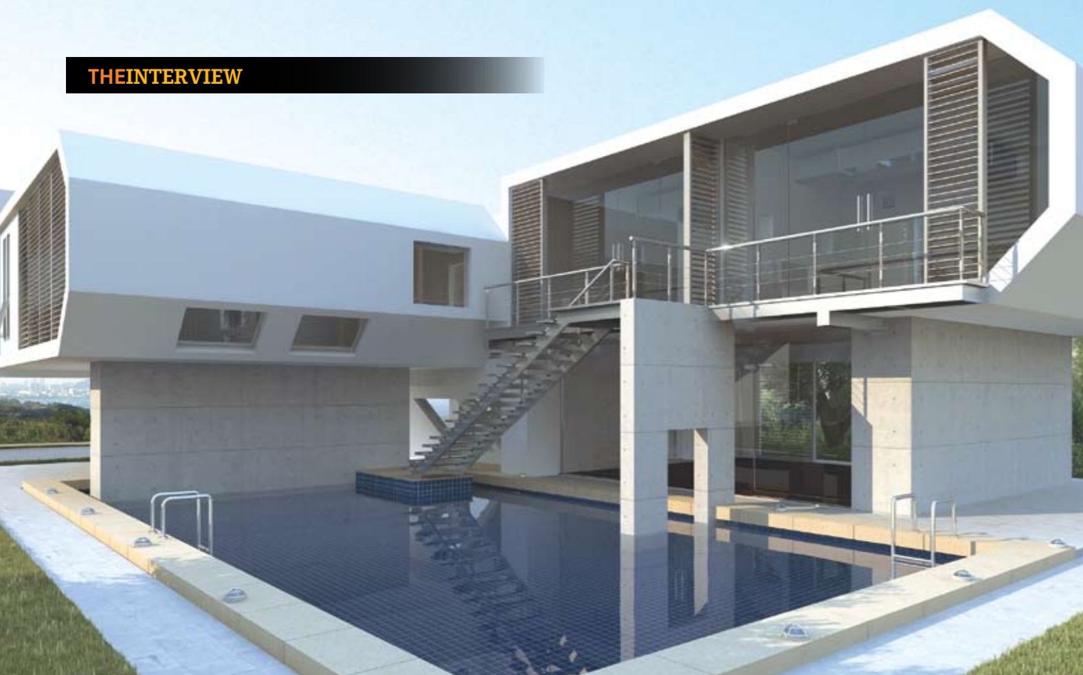
Capson: A Japanese house on Pratamnak Hill for a Danish client. A cube or capsule design – hence its name – this house is of pre-cast concrete with no interior bars or columns, blue reflective UV glass, a heavy-duty aluminium frame, blue reflective pool tiles, tropical woods and stainless steel. Finished in white concrete, the house is another example of extreme engineering with 55 degree walls containing windows overlooking the pool. It also features an industrial, heavy-duty air conditioning system.
