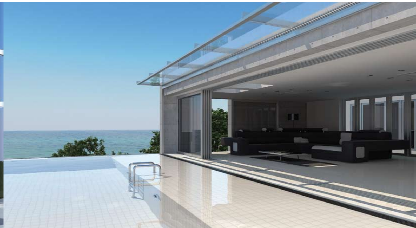
Merit Villa: Located at Wongamat, this house has been designed for a German client and features pre-cast concrete, steel beams, green reflective UV glass, a heavy-duty aluminium frame and tropical woods. Finished in white concrete, the villa has large spans and no columns, a white tiled swimming pool and an underground car park.
